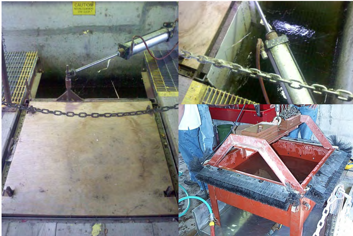
Figure 2. Adult trapping facility at Rocky Reach Dam. The pneumatic arm (left and top right) activates a gate that guides fish into a holding vessel (bottom right, shown lifted). Trapped fish are either allowed to exit the holding vessel by opening the gate, or are lifted for processing.
