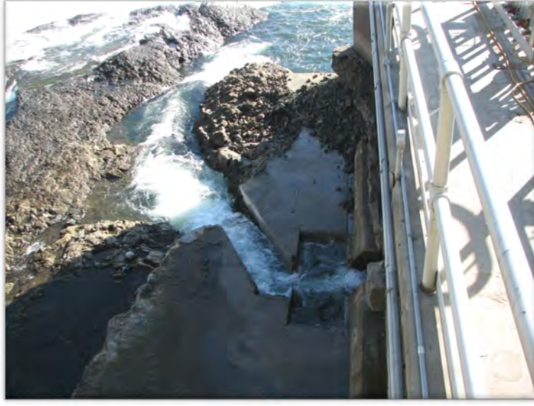
Photo: Rock Island center ladder side entrance modification.
