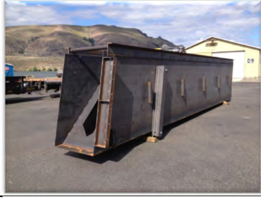
Photo: Staging of the denil for the left bank fishway entrance extension.
