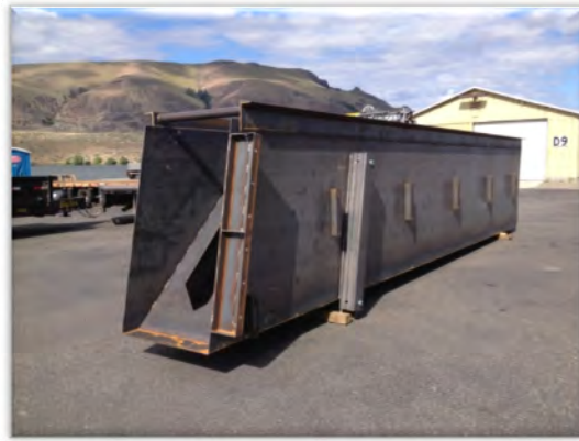
Photo: Staging of the denil for the left bank fishway entrance extension.
