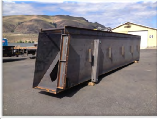
Photo: Staging of denil for the left bank fishway entrance extension.
