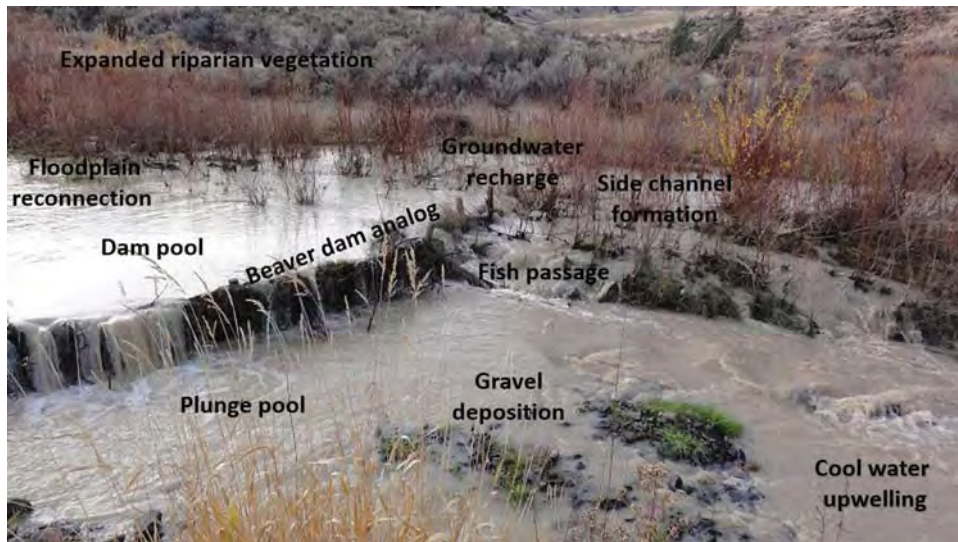
Figure 3. Example of a beaver dam analog (BDA) annotated with some of the expected responses.
