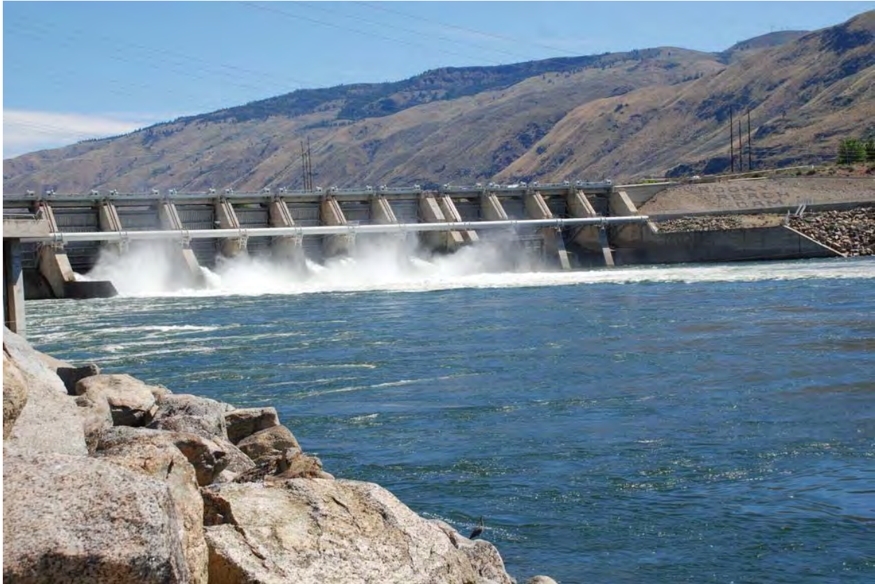
Figure 3. Rocky Reach Project spillways.
