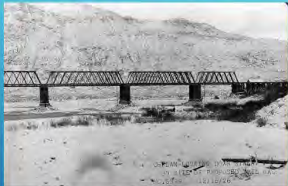
Looking downstream on site of proposed tail race, 12/15/26
