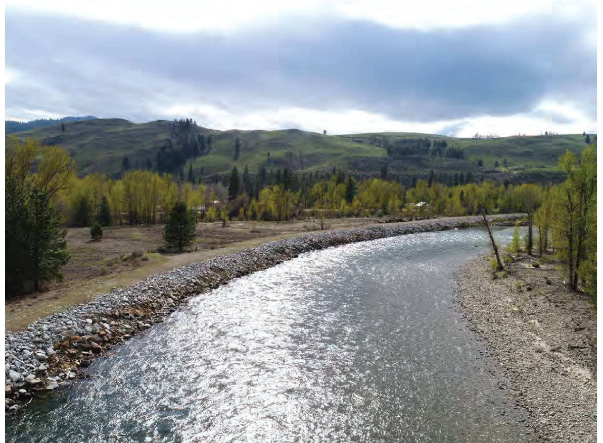
Levee – looking upstream toward Hwy 20
