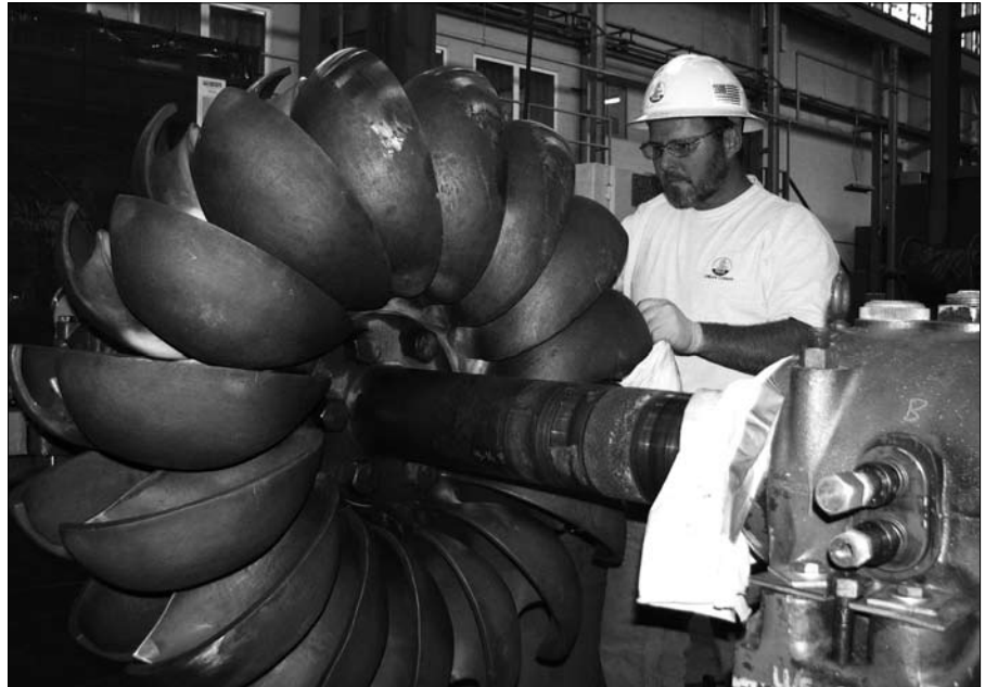
Journeyman Mechanic Jack Brown inspects the Stehekin power plant's refurbished Pelton wheel. The repaired wheel, or turbine runner, has been placed back in service temporarily until a new runner can be cast.
