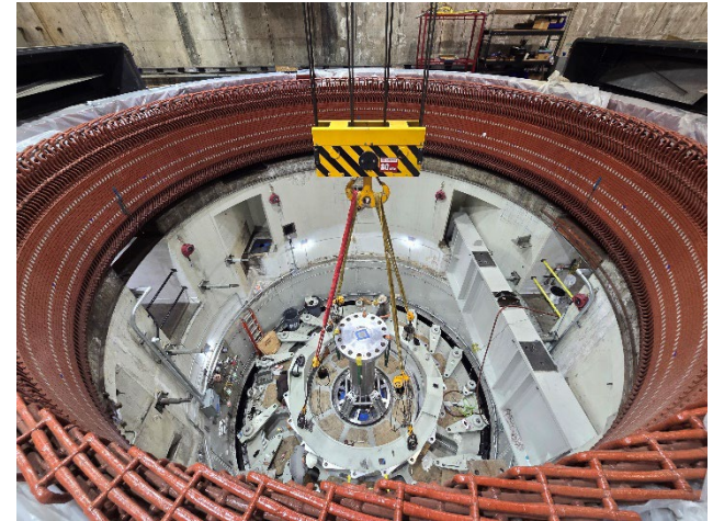
Rock Island PH1 Modernization Est. Completion: 2028
